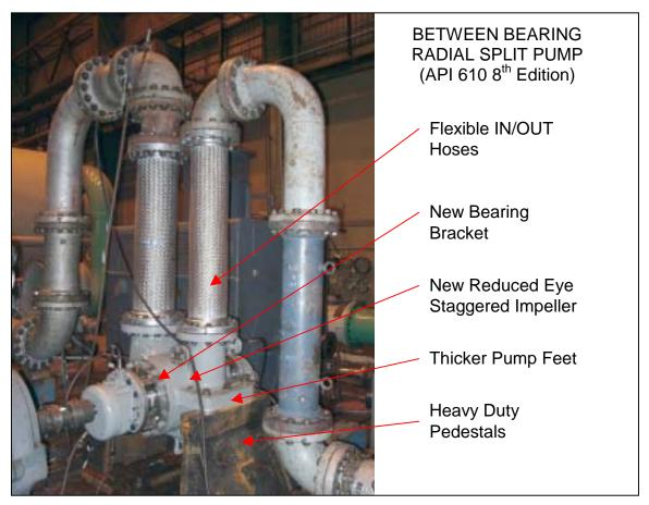
Figure 1 Vibration Reducing Test Loop
