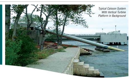
Flowserve submersible incline pumps are a proven reliable and cost-effective alternative to vertical turbine pumps for lake, river, open-pit mine and quarry pumping applications. Unlike the vertical turbine pumps, the submersible incline pumps do not require building a structure for operation.
