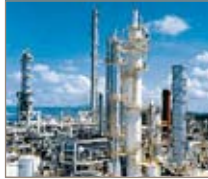
Figure 6 – A Post-Combustion CO 2 Capture Unit Source: [1]
