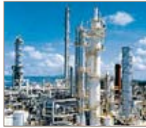
Figure 6 – A Post-Combustion CO 2 Capture Unit Source: [1]
