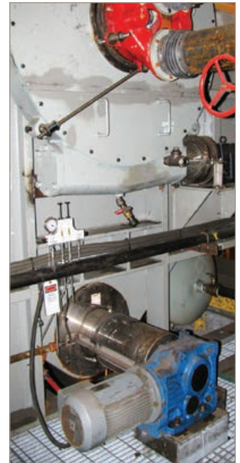
Figure 3: Plant area after the seal retrofit
