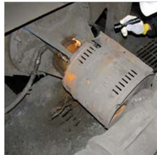
Figure 2: Plant area before the seal retrofit
