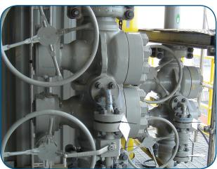
The valves illustrated are 6" class 2500 with hub ends, in carbon steel, manually operated.
