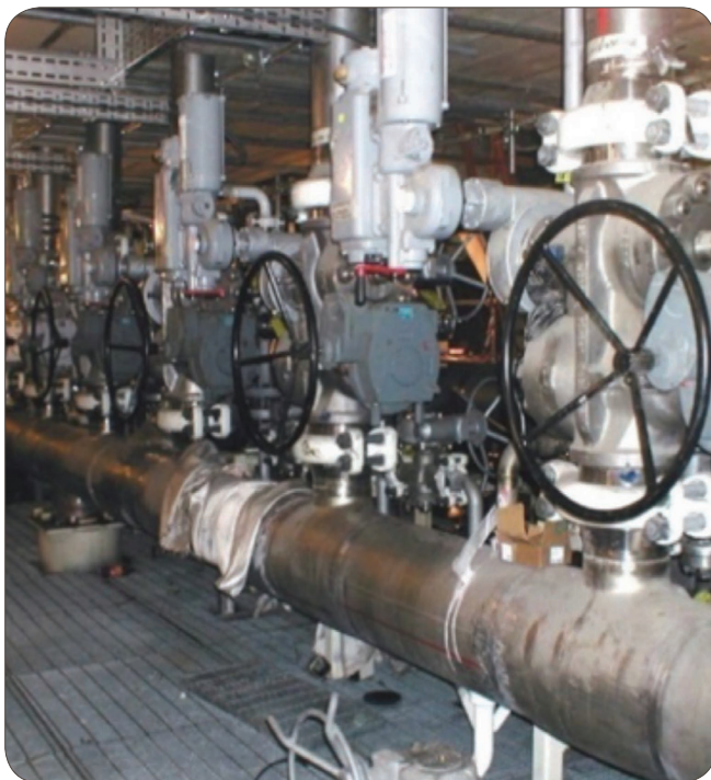
Figure 1a: Offshore manifold with DB&B plug valves
