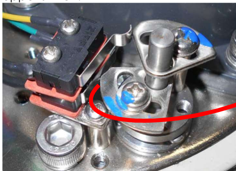
Figure 12: The lower cam is tripping the lower switch.
