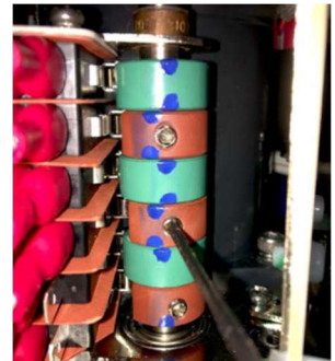
Figure 26: Cam 3 and cam 5 (CW auxiliary switch cams, red)
