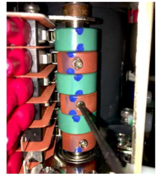
Figure 11: Cam 3 and cam 5 (CW auxiliary switch cams, red)
