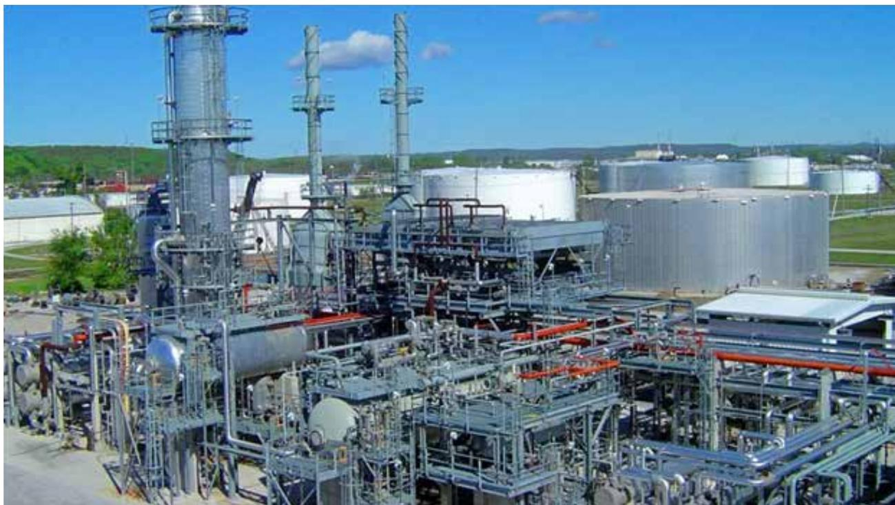
**Hydrotreating** is the process for removing objectionable elements from products for feedstocks by reacting them with hydrogen in the presence of a catalyst. The objectionable elements include sulfur, nitrogen, oxygen, halides and trace metals. Hydrotreating is also referred to as hydrodesulphurization, or HDS.
