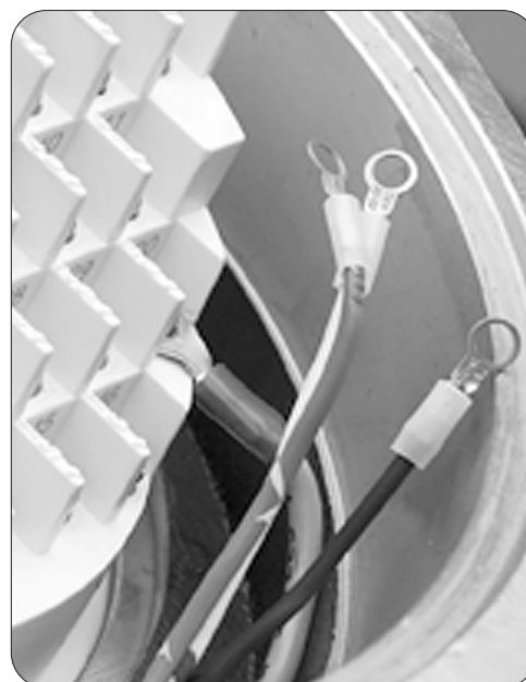
Figure 3.14: Stripping conductors and applying heat shrink tubing
