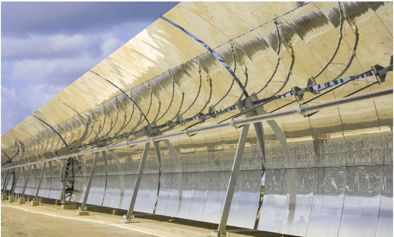
Figure 1: Parabolic trough mirror and receiver
