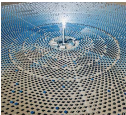
Figure 2: Tower or central receiver
