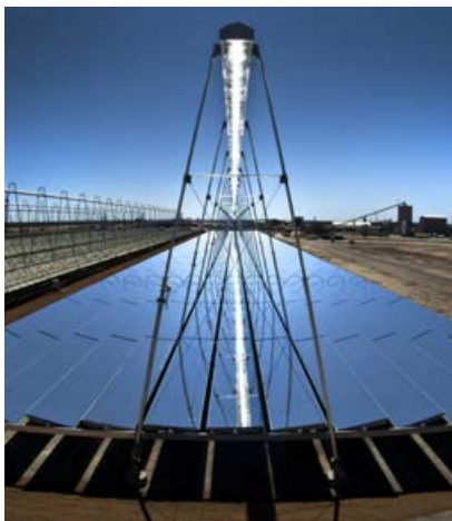
Figure 3: Fresnel mirrors and receiver
