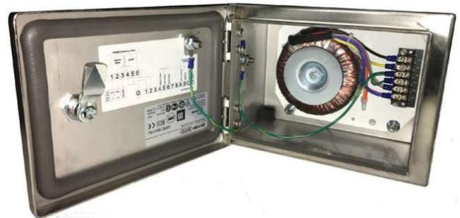
Figure 11: LTQ Series Transformer (120/230VAC Installations)
