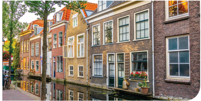
Dutch home might soon be warmed by lower-cost heat from Gasunie's WarmtelinQ heat grid project. By repurposing waste heat from industrial plants near the port of Rotterdam, WarmtelinQ will support a cost-effective alternative to burning fossil fuels and reduce CO 2 emissions.
